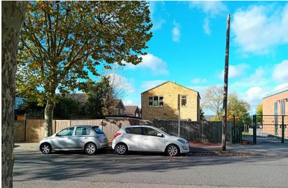
Figure 3 – Front elevation of School House
